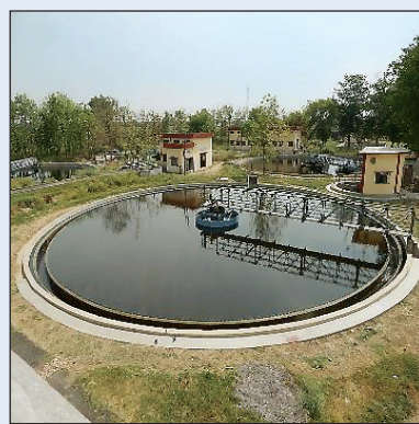
Treatment Plant, Allahabad
