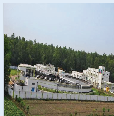
Treatment Plant, Haridwar
